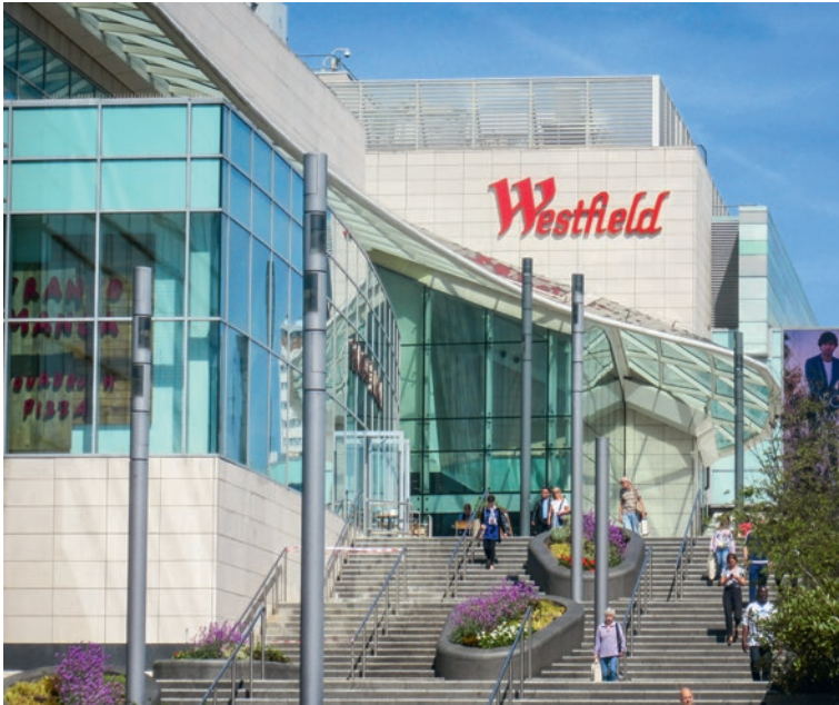
Westfield, Shepherd's Bush: works to extend the shopping centre had to be kept separate from the existing structure
