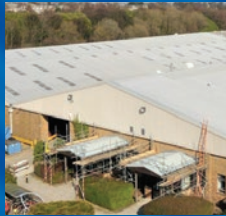
Lightweight GRP over-roofing Water company depot, Yorkshire
