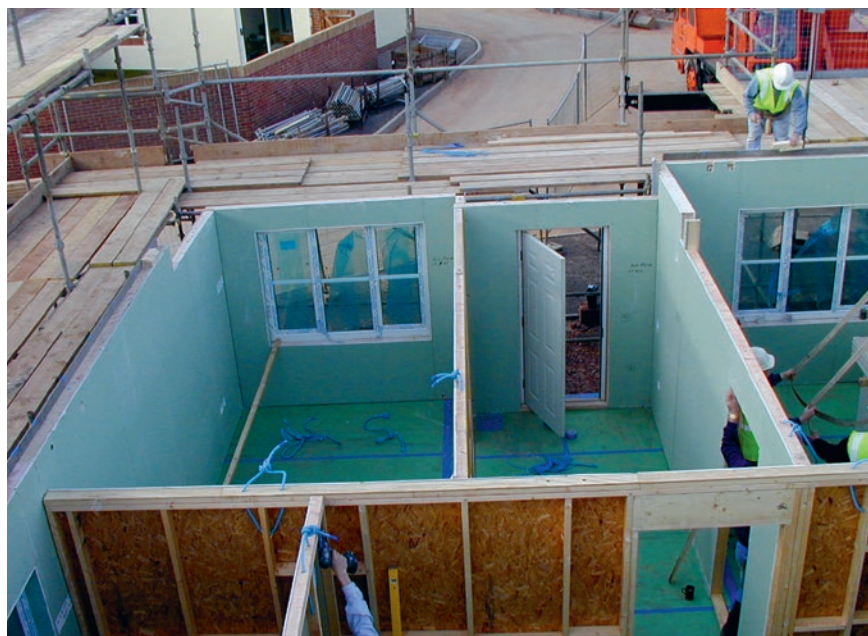
Assembling a house that has been manufactured off site: housebuilders are investing more in modern methods of construction, partly in response to skills shortages
